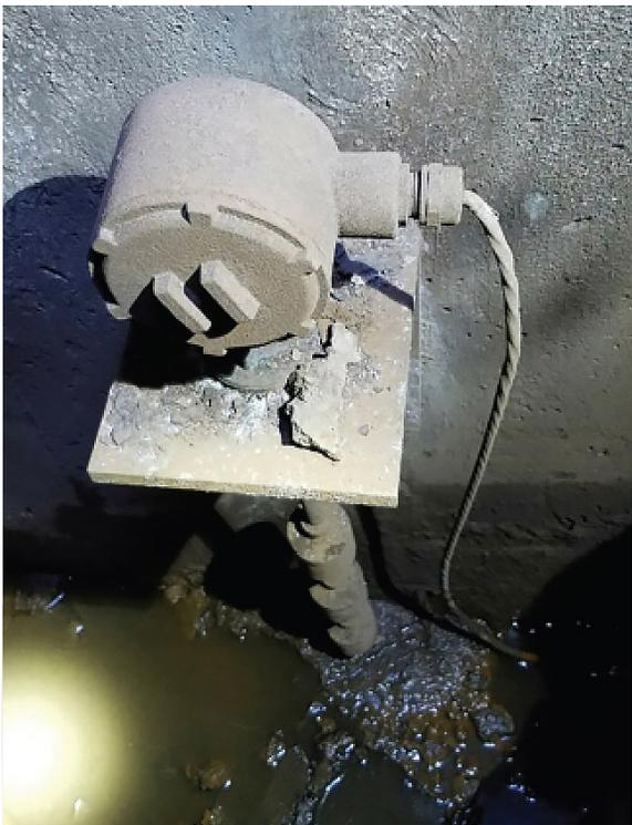
Float switches can be constructed of different materials to withstand chemicals, high temperatures, high pressures, and even acidic environments. They are suitable for fluids that remain liquid well below freezing, and for high-temperature applications like hot oils to 482F/250C.
